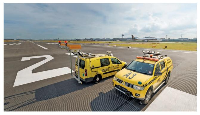
To combat the projected future increase in heavy rainfall, CAG has grooved the asphaltic pavements of all three runways at Changi Airport to reduce the danger of aquaplaning and runway excursions on wet surfaces during thunderstorm events.
